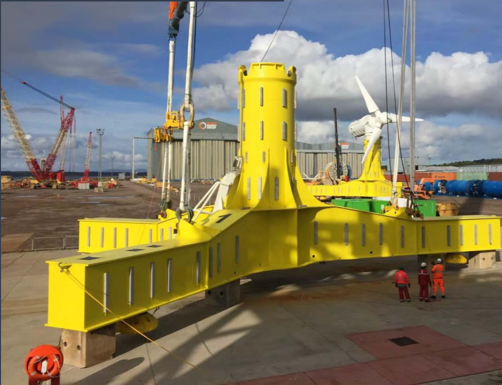
Foundations constructed and ready for load out
